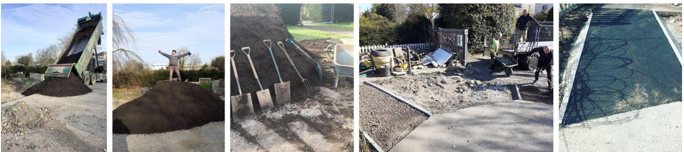
Feb 2021 - groundwork, new pathways and topsoil delivery
